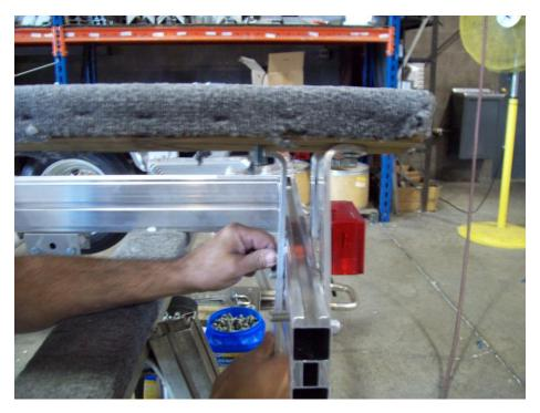
After you install the outside bunk boards go back and add the slotted angle brackets to front of each board as shown. Final adjustment will be made when boat is on the trailer.
