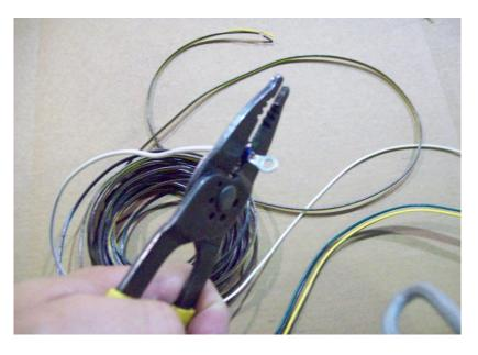
Cut the white ground wire at 31" from the connector. Strip the ground wire and install ring terminal.
