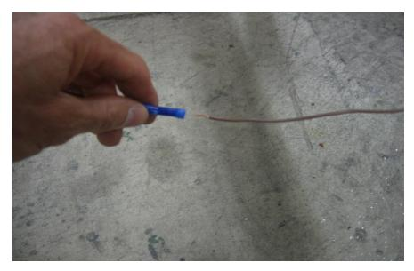
Use the left over brown wire and strip <sup>1</sup>/<sub>4</sub>" of insulation from the end. Install a butt connector by crimping it onto the bare wire.
