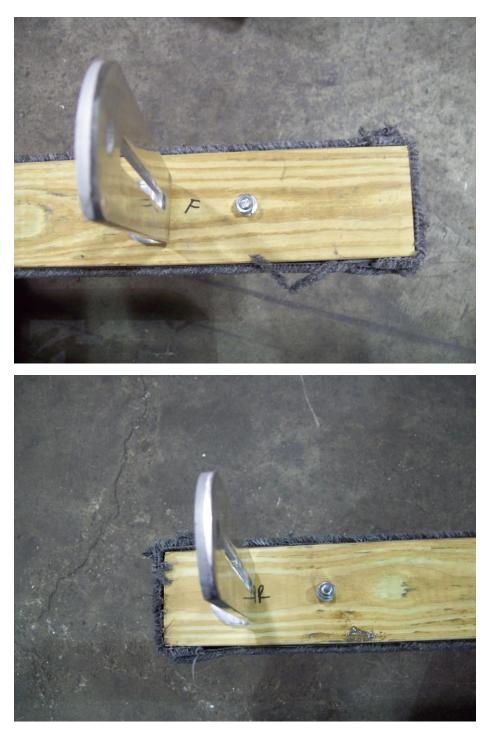
Install the slotted angle brackets to the front and rear of the bunk boards as shown.
