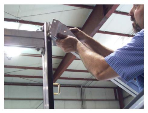
Install the right side top offset attaching plate.
