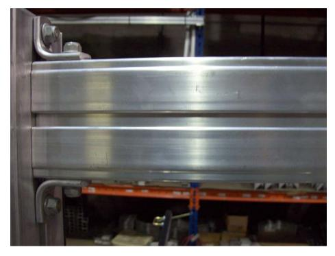
Position the top of both angle brackets on the horizontal bar even with the top of each vertical post.
