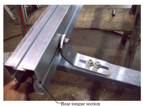
First install the rear cradle bracket and slide forward for now.
