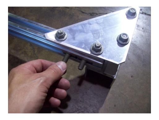
Install 2 T-bolts to the front side of the forward cross member.
