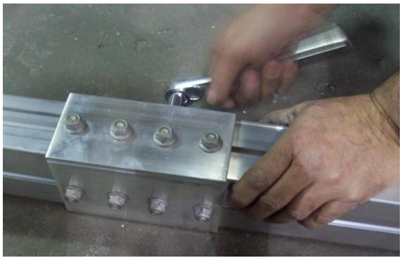
Slide bottom plate over and align with side plates. (bottom of tongue)
