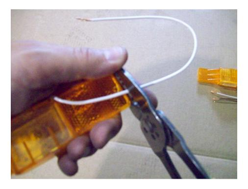
Cut approximately 8 ½" off of the white wires on both running lights.
