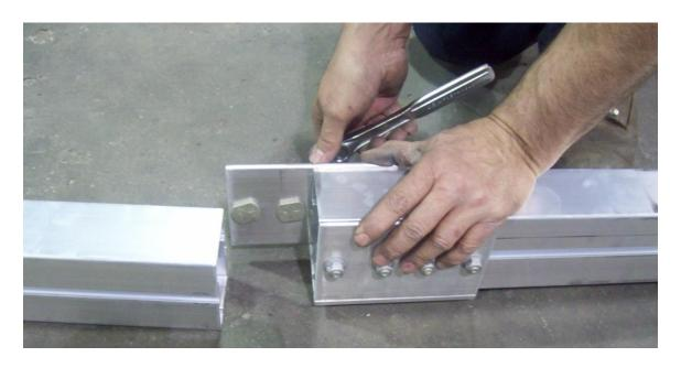
Center one side splice plate and tighten.
