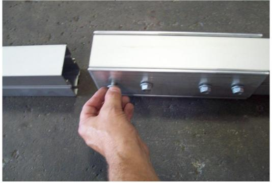
Unwrap the two tongue sections and install four T-bolts on the rear section on each side. Then add splice plates and nuts.
